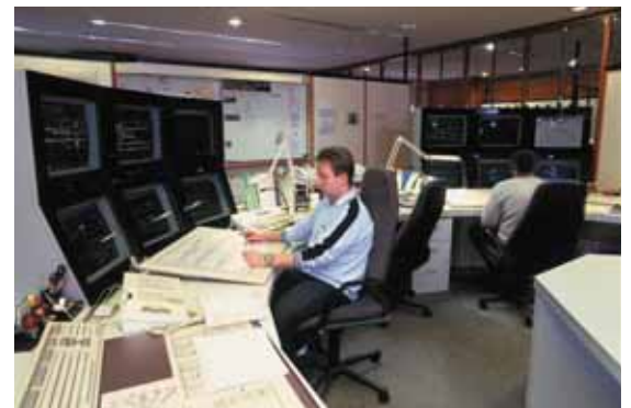
3 Siemens-built S-Bahn transit operating center in Berlin
