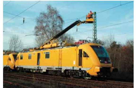
2 Modern maintenance vehicle built in Kirchmöser
