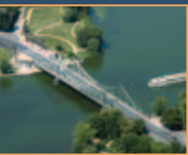
Glienicker Brücke – linking Berlin with Potsdam
